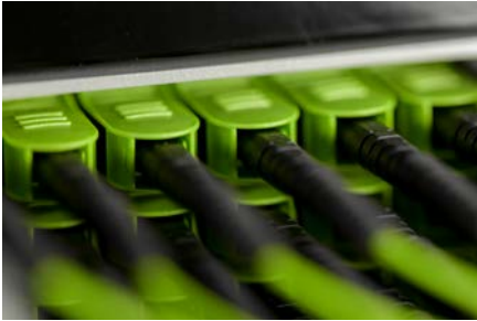
041.0312 OM5 LC-QR ports in Netscale 120 platform
